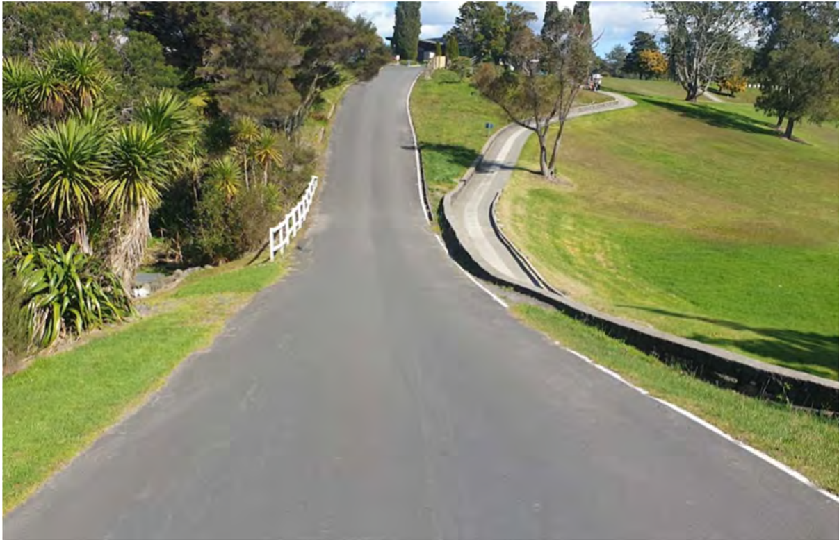
Figure 2 – Road Low Point
